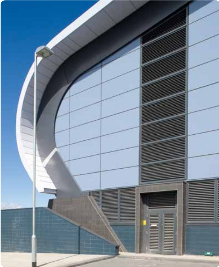
Ref. Sunderland Aquatics Centre, Sunderland (UK), Arch. Red Box Architecture
